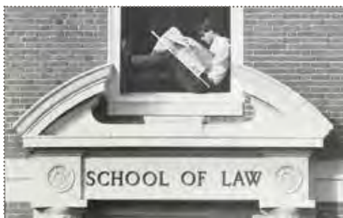
Above: Carswell Hall under construction. Left: A student reads a newspaper in the window above the entrance to Carswell Hall.
