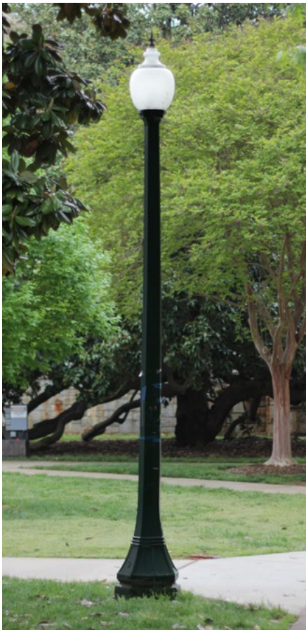
fig. 02f: SITE LIGHTING - ACORN PEDESTRIAN POLE
