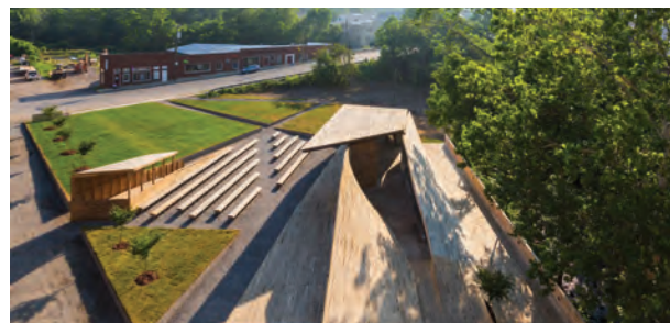
Masonic Amphitheater Project Clifton Forge, Virginia
