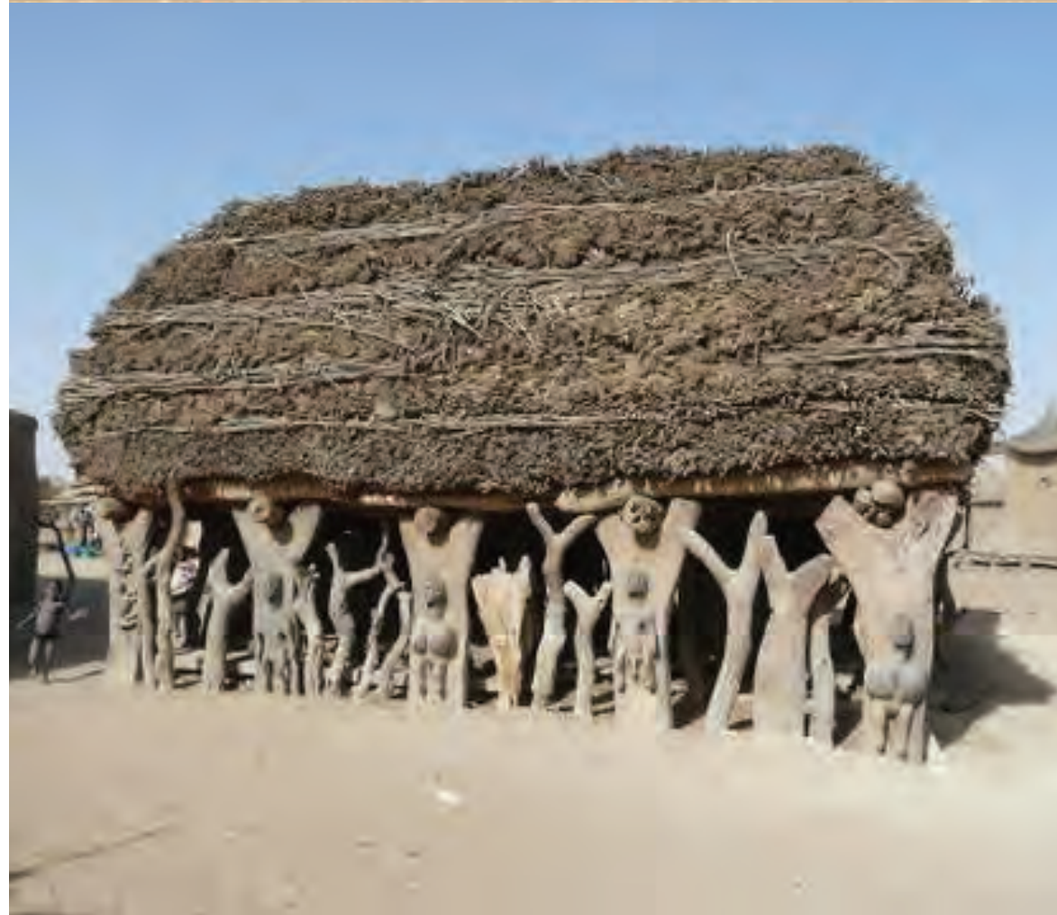
Toguna with many Kile Wood posts Various Vernacular Builders Dogon Country, Mali
